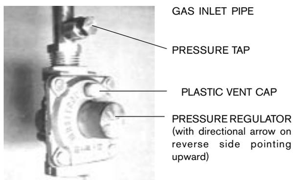
**Fig. 5 - Installation of Gas Pressure Regulator**
