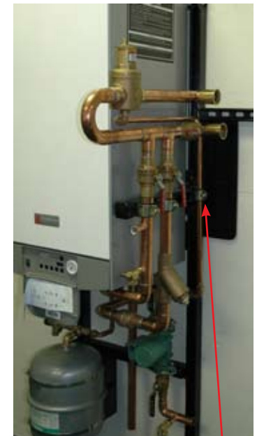
Secure fill water line with strut clamp
