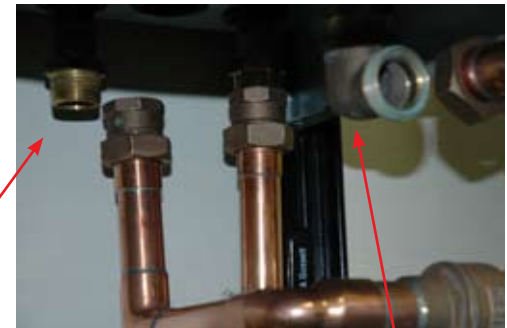
Screw 90 degree half union on supply port, make sure it points to the front
