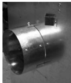
Center Round Duct collar over hole and attach to the tabs using 3 screws
