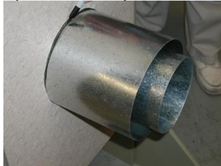
Step 3 – Mark 8” Protection Pipe at Inside Wall
