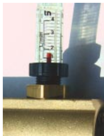
Fully open balancing valve
